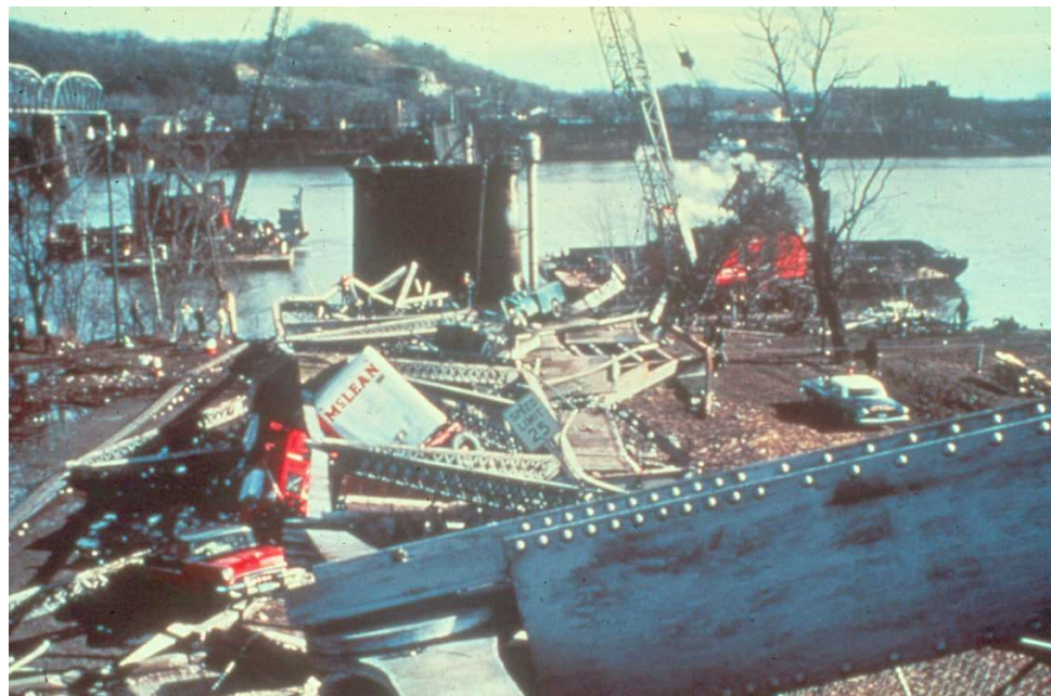
Figure 1.1.2 Collapse of the Silver Bridge
