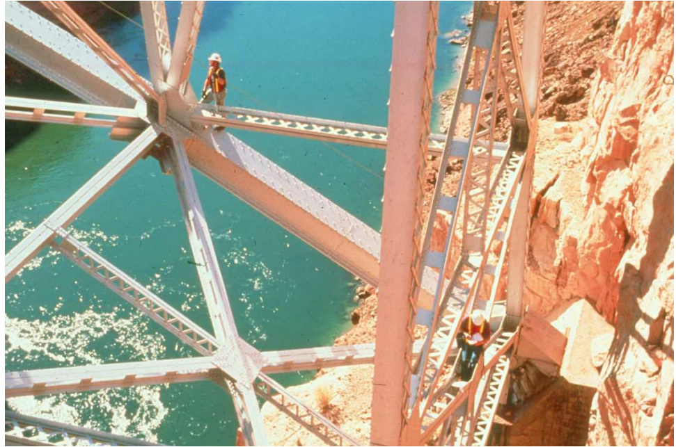
Figure 2.2.7 Inspection Involving Extensive Climbing
