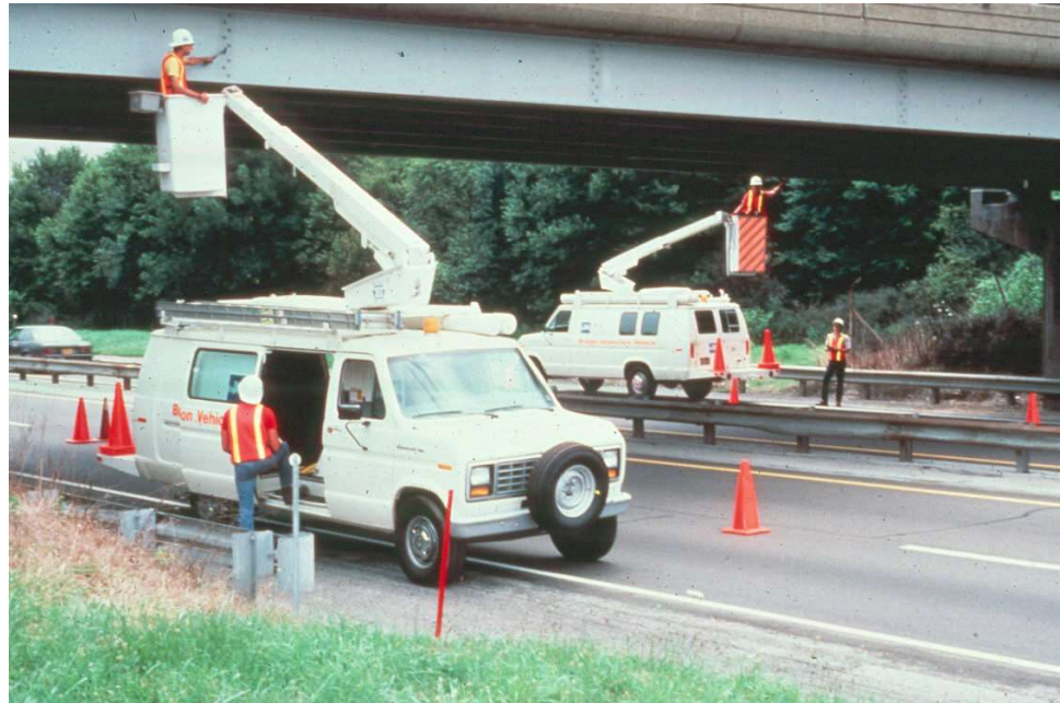
Figure 2.3.3 Inspection Vehicles with Flashing Light
