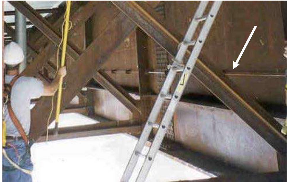
Figure 2.5.13 Handrail on Girder Bridge
