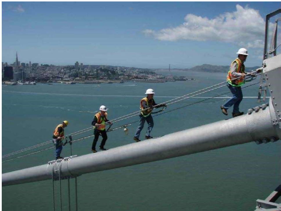
Figure 2.5.14 Handrail on Suspension Bridge
