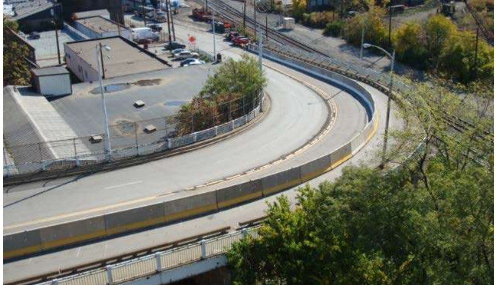
Figure 2.3.13 Temporary Traffic Barriers
