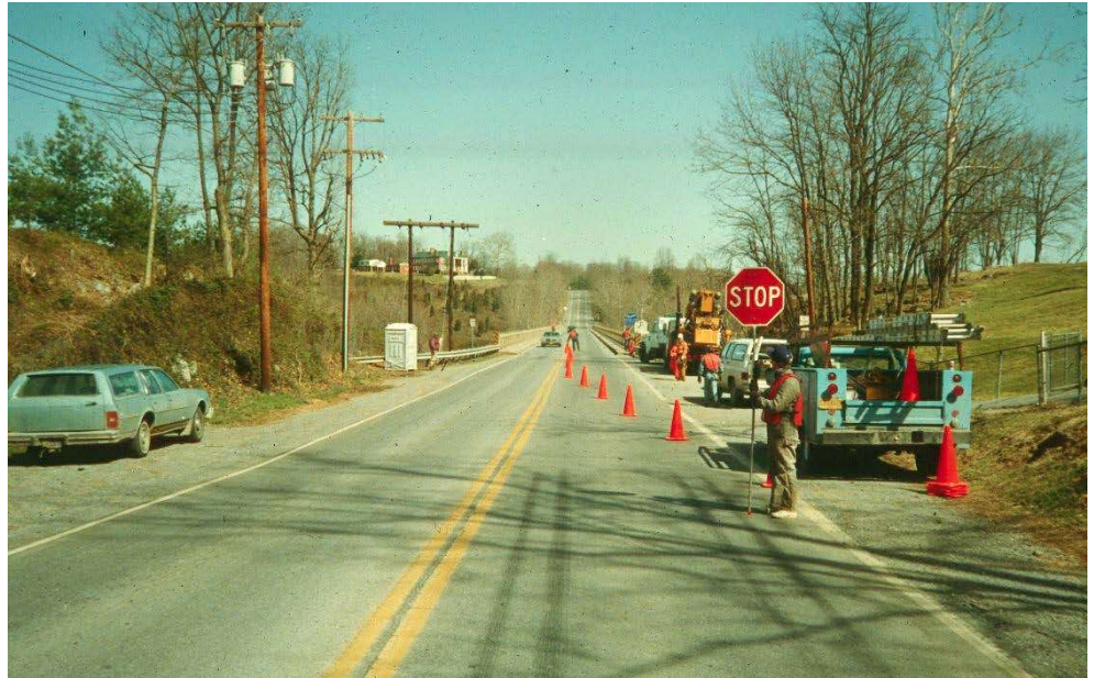
Figure 2.1.4 Temporary Traffic Control Operation
