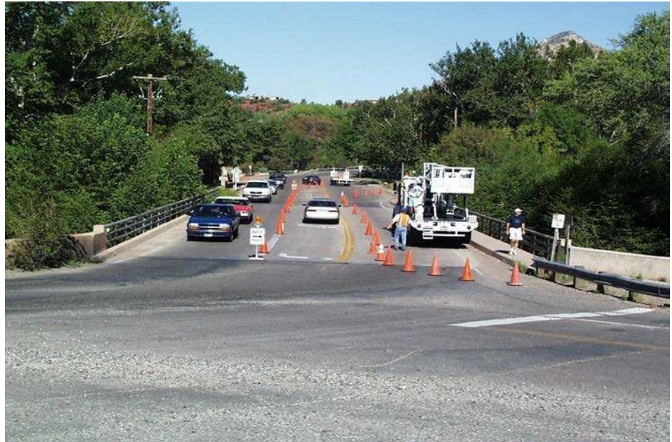
Figure 2.3.1 Temporary Traffic Control Operation
