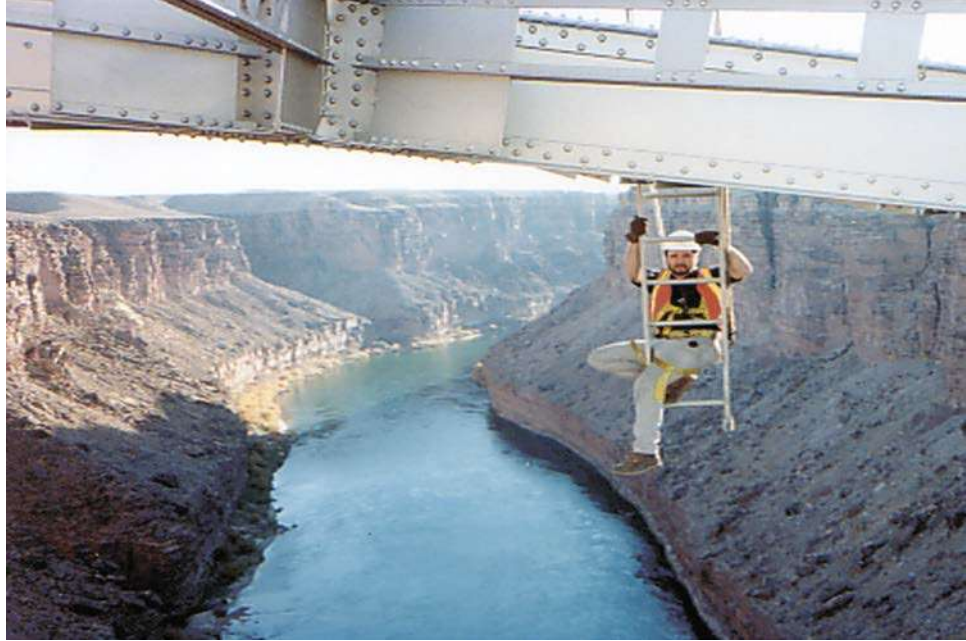
Figure 2.5.2 Inspector using a Hook-ladder
