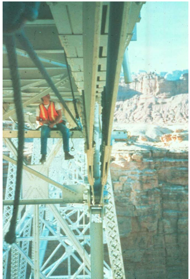
Figure 2.5.4 Rigging for Superstructure Inspection
