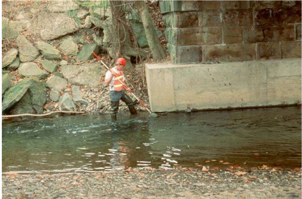
Figure 2.1.5 Inspection for Scour and Undermining
