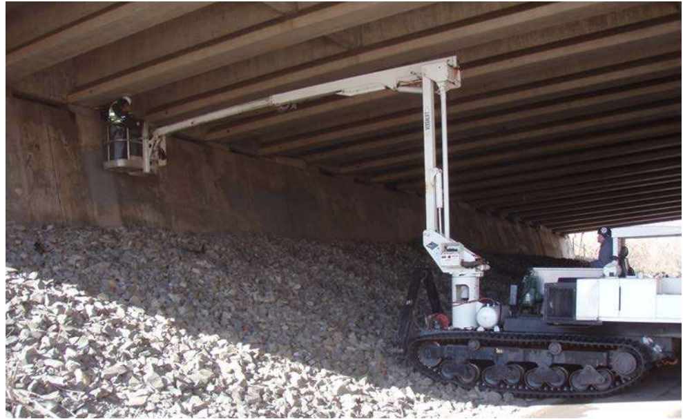
Figure 2.5.19 Track-mounted Man-lift on a Slope
