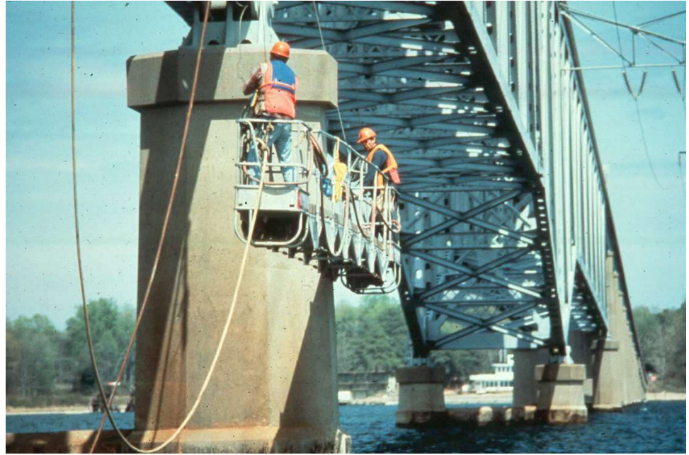
Figure 2.5.3 Rigging for Substructure Inspection
