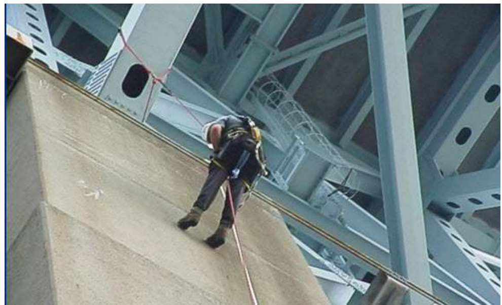
Figure 2.5.9 Inspector Rappelling Substructure Unit
