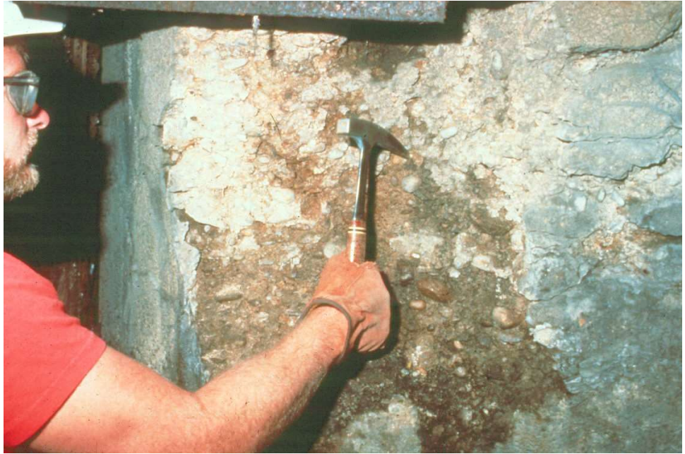
Figure 2.2.3 Inspector Wearing Safety Goggles and Gloves
