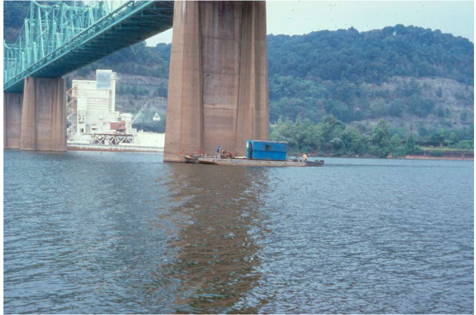
Figure 2.5.6 Inspection Operations from a Barge
