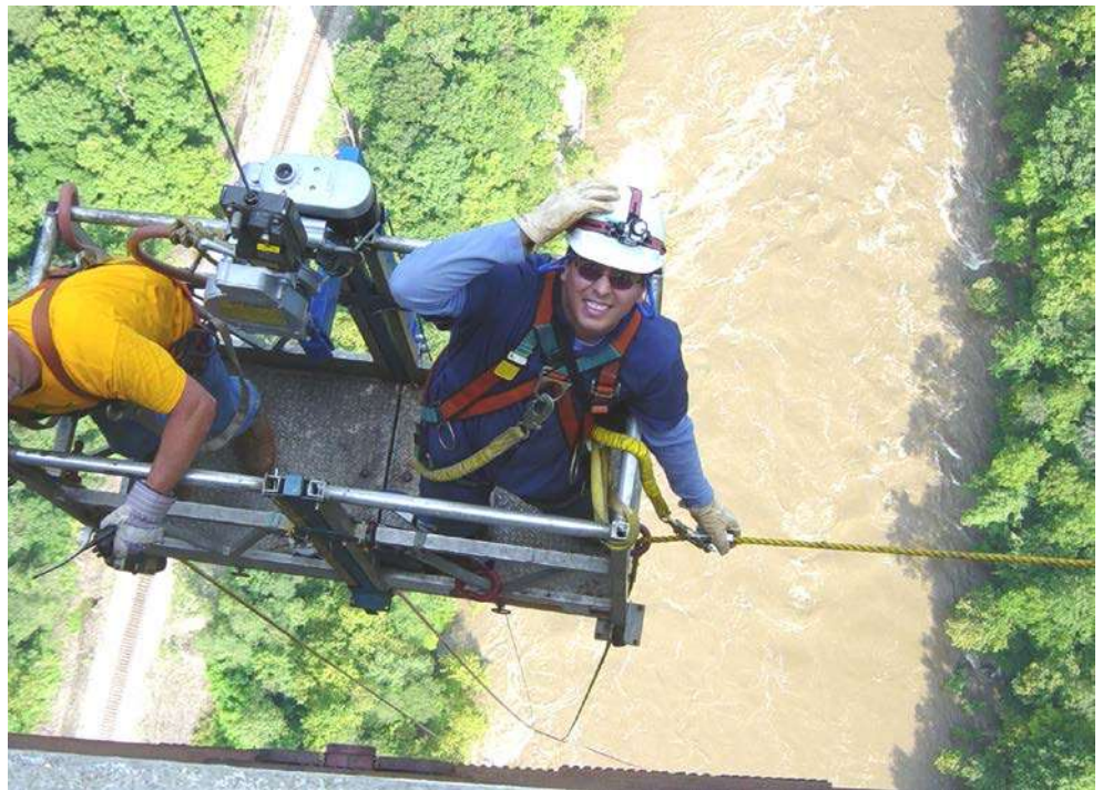
Figure 2.2.6 Inspector with Safety Harness with a Lanyard
